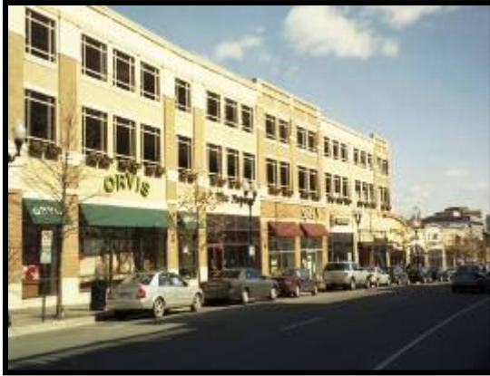
Parking Ramp Above Retail
